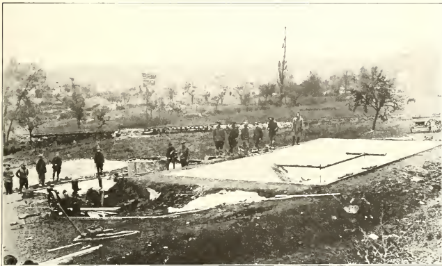
A FILTRATION PLANT A FEW KILOMETERS FROM THE FRONT — AT EUVEZIN. OCTOBER 22, 1918.
